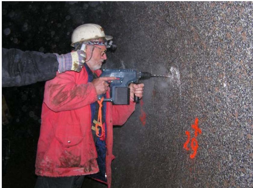
Fig. 4: Preparing for fixation of geophysical sensors (geophones, electrodes).
