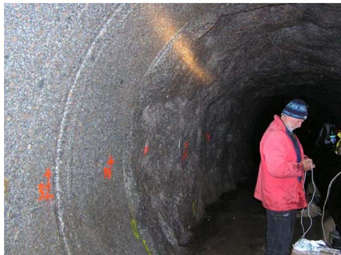
**Fig. 2: Look on the gallery (interface between machine-driven and hand-driven parts of the tunnel).**
